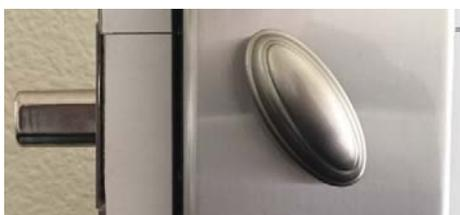
The turnpiece (also known as a tailpiece) is the portion of your lock that extends through your door from the outer key cylinder to the inside of your door. The thumb latch connects to turn piece in order to operate your lock. Your Lark-Wi lock will attach to this in place of the thumb latch.
